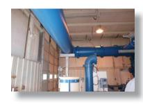
The Chemical Feed Building Expansion project includes enlarging the existing chemical feed building, supplying new bulk coagulant and polymer feed system pumps and piping and lighting, heating and electrical improvements. The design of this portion of the project began in April 2011.
