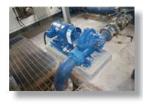
This project consists of two parts: the Water Plant High Service Piping and Booster Pump Station Improvements and the Chemical Feed Building Expansion. The Water Plant High Service Piping and Booster Pump Station Improvements included increasing the size of the high service piping from 12" diameter to 24" diameter and replacing several motor control valves. This project also included replacing pumps and pump pads at two separate booster pump stations located on the distribution system.
