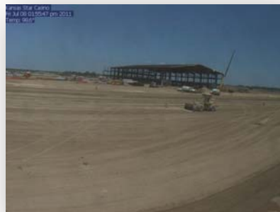
On-going construction; obtained from www.kansasstarcasino.com
